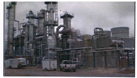
Two new evaporators have been installed at the Pratt Energy plant.
